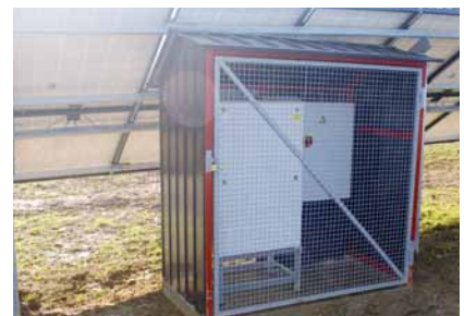
Weatherproof: The inverters of the SolarMax S series can be installed inside and out – even for this freestanding system in Gornji Petrovci.
