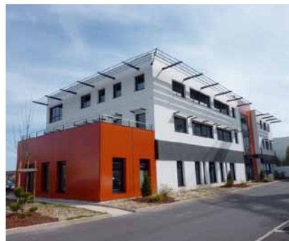
Equipped for further growth: The new company headquarters of Sputnik's French branch office in Saint Priest near Lyon.
