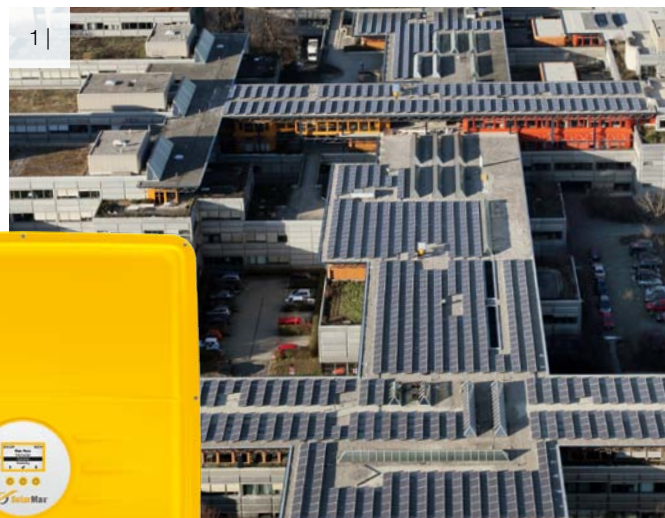
1 | Photovoltaic plant at the EPFL university campus in Lausanne – the largest solar power plant in Switzerland with 42 SolarMax MT inverters
