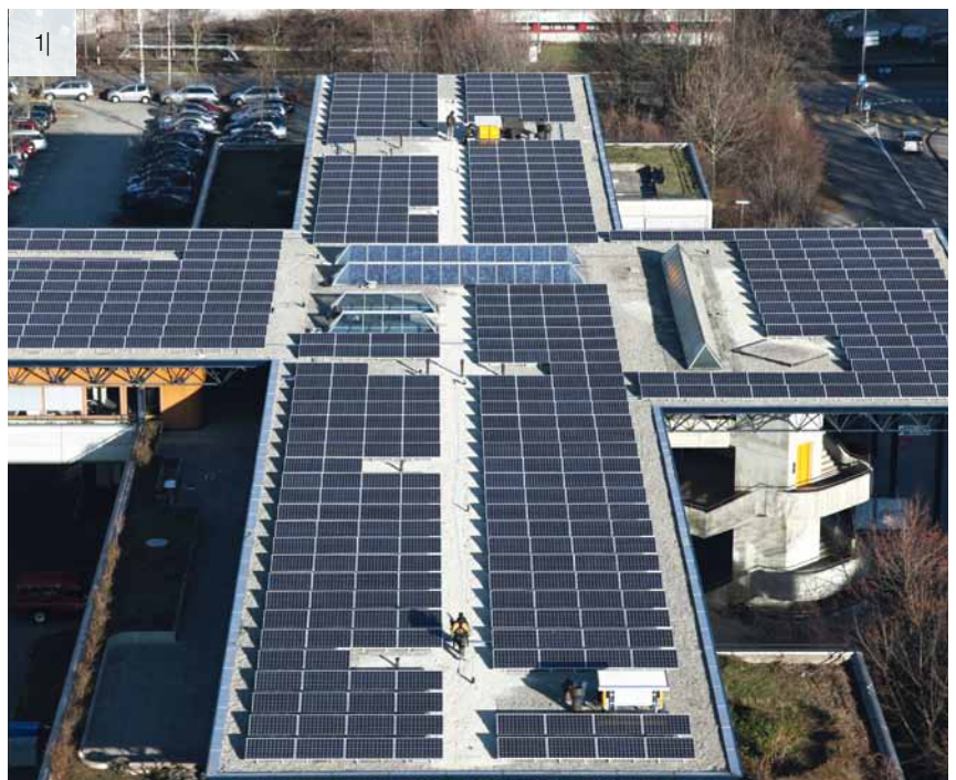
1| In the first phase of the plant Solstis installed monocrystalline modules on flat roofs. By fall 2012, building-integrated systems and dye cells will follow on the EPFL campus.
