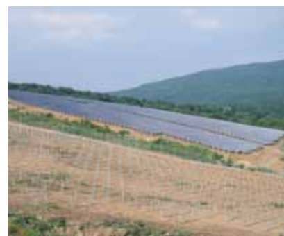
Bulgarian investment: Solar power plants are especially attractive. Here is a 2-megawatt system in western Bulgaria.
